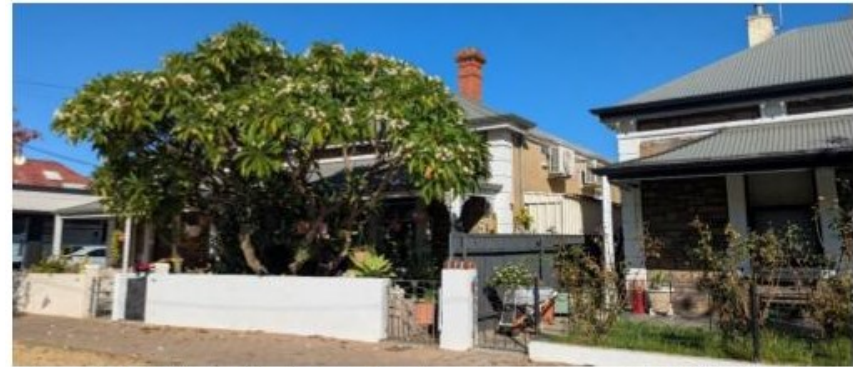
Figure 32: Semi-detached dwellings continue the scale and form of nearby Halifax Street houses Source: CGA, 2025.
