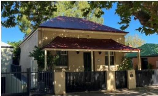
Figure 23: 47 Stanley Street Source: GCA2025
